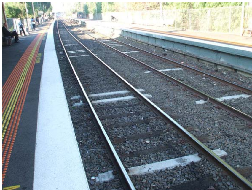
Figure 4.9 Old timber sleepers being replaced by concrete sleepers to resist track buckling
