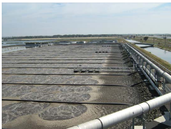
Figure 4.15 ASP aeration basin
