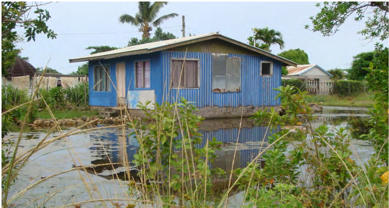
Figure 1: High tide in the village of Popua, on the eastern fringe of Nuku'alofa, Tongatapu, where families are reclaiming land to build (Photo: Neal Smith)
