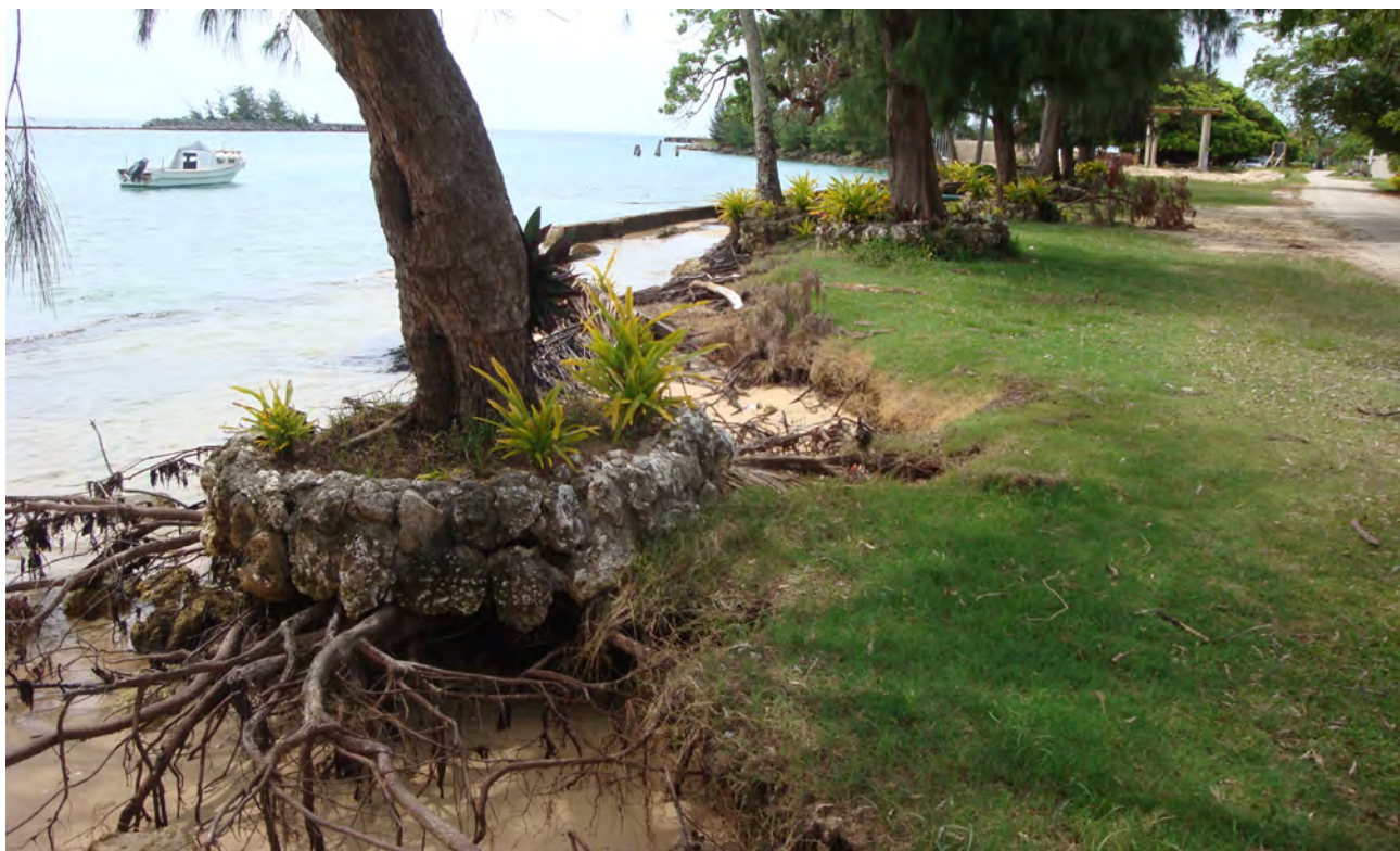
Figure 5: Coastal erosion at Lifuka
