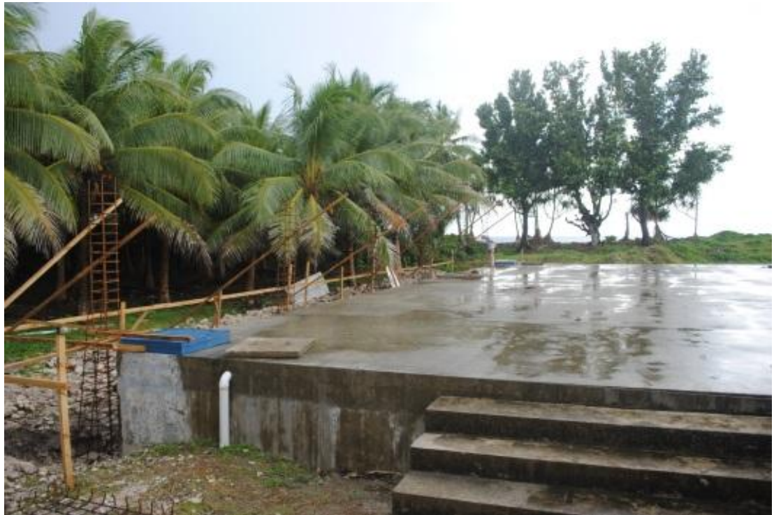
Figure 12: A 750 kL cistern under construction in Lofeagai village, Funafuti
